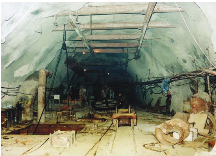
Figure 5. Underground workings at the Mecsek Uranium Mines.
